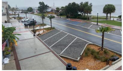
Permeable Pavement & Bioretention (St. Marys)
